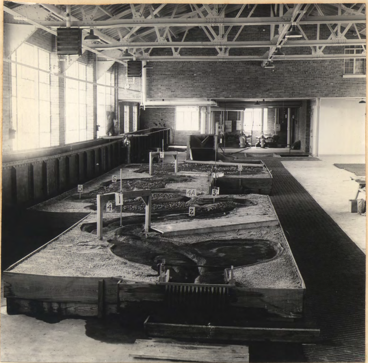
PLATE I. GENERAL VIEW OF THE GREENVILLE BENDS MODEL, U.S. WATERWAYS EXPERIMENT STATION, VICKSBURG, MISS. MODEL SCALES: 1:4800 HORIZONTAL, 1:360 VERTICAL.
